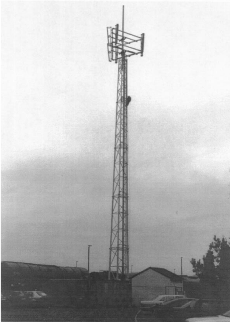
Figure 1. Steel transmitter mast with eccentric antennae at the top.
