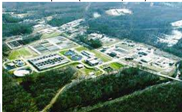
Figure 2: Aerial view of the North and South Durham water treatment facilities (Hazen and Sawyer)
