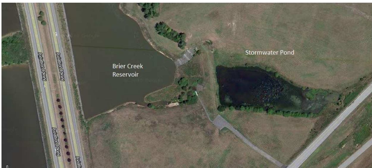
Figure 3. Another example of an RDU Stormwater Detention Pond (from Google Maps)
