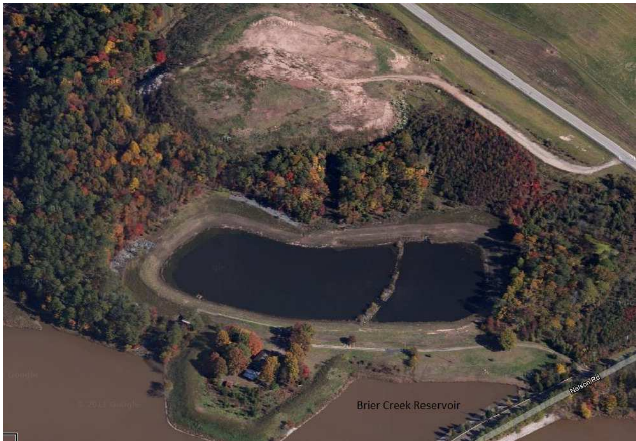
Figure 2 - Completed detention pond next to reservoir (from Google Maps)
