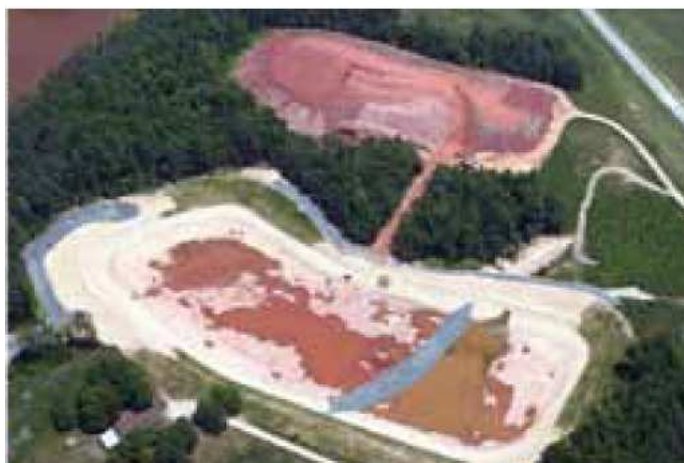
Figure 1 - Construction of detention pond next to reservoir (Parsons 2005)
